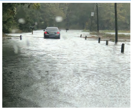
A car approaches a flooded section of Old Quarry Road in Guilford during a nor'easter in October 2018. The road had been raised about two feet within the last three years, but continues to flood during storm events. Photo: Sidney Gale
