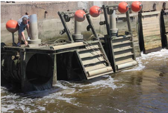
The self-regulating tide gates installed on the West River five years ago allow salt water to flow upstream, restoring a tidal marsh and reducing flooding in the surrounding area.
