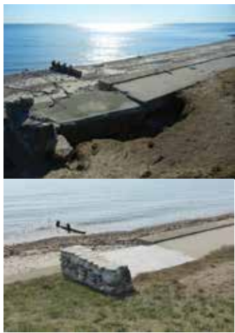
Sandy’s damage to a seawall in Old Saybrook is seen here before and after repair. Photo credit: Juliana Barrett.
