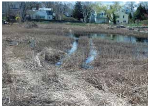
Taken in May of 2014, this photo illustrates the extent of invasive species debris removal that was necessary prior to the first planting stewardship events. Photo credit: Beth Sullivan.
