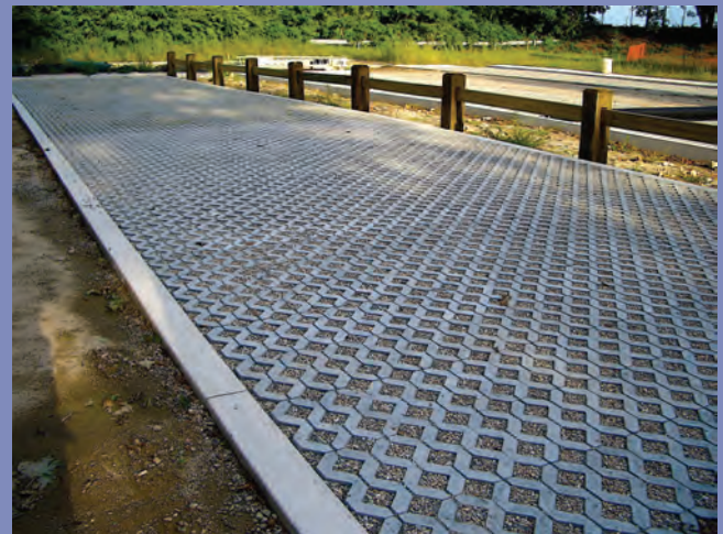
Low impact design includes the use of porous pavement that permits rain water to infiltrate into the ground. Photo Judy Preston
