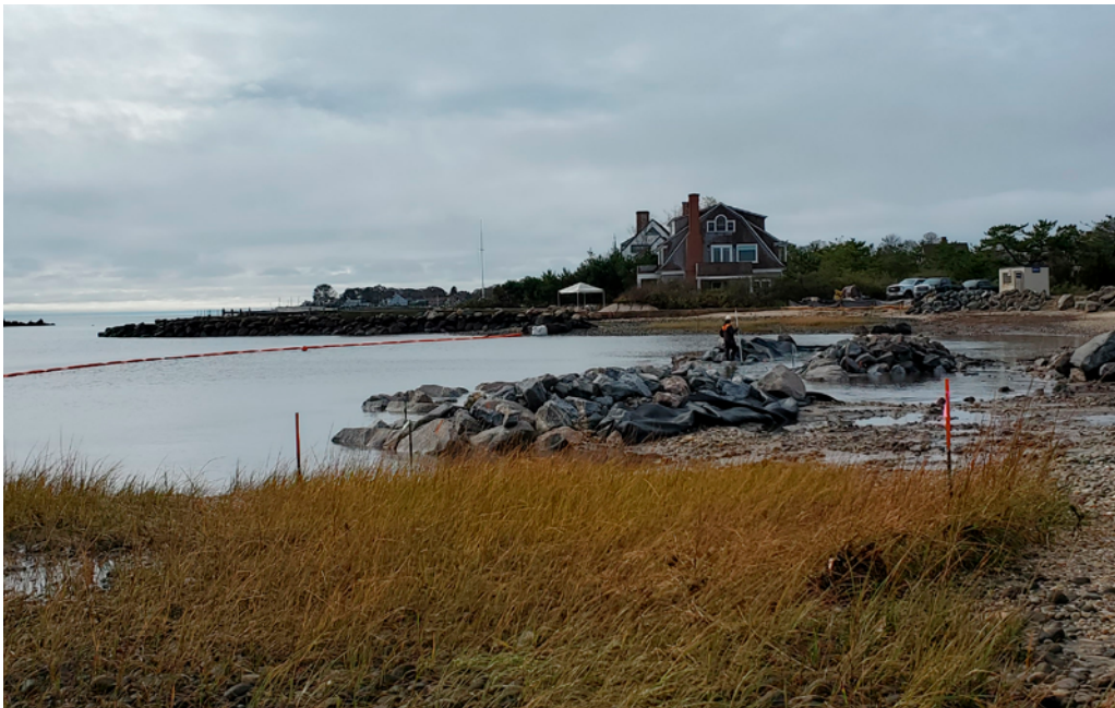
FIGURE 5.11 Completed rock sill along coastline of Fenwick Point in Old Saybrook. Photo: Juliana Barrett
